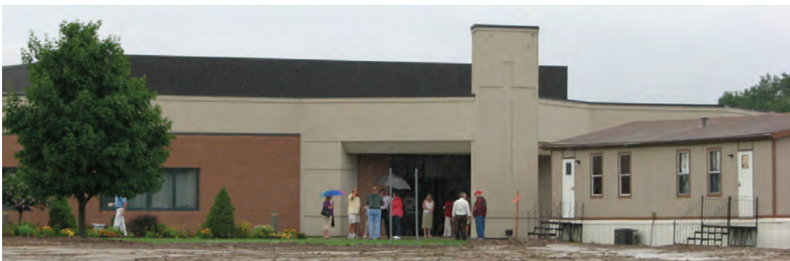
The current facilities at Alive in Christ, Columbia. The new construction will eliminate the need for the portable classrooms (right).
